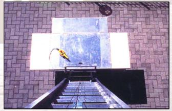
All ladder elements are made of aluminum EN AW-7020 designed for very light structures with maximum load capacity of 250 kg.
